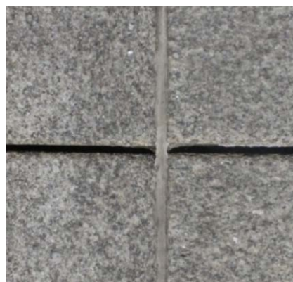
Figure 5. Example of dilatation joint in good condition (vertical), grout joint with some damages (horizontal).
